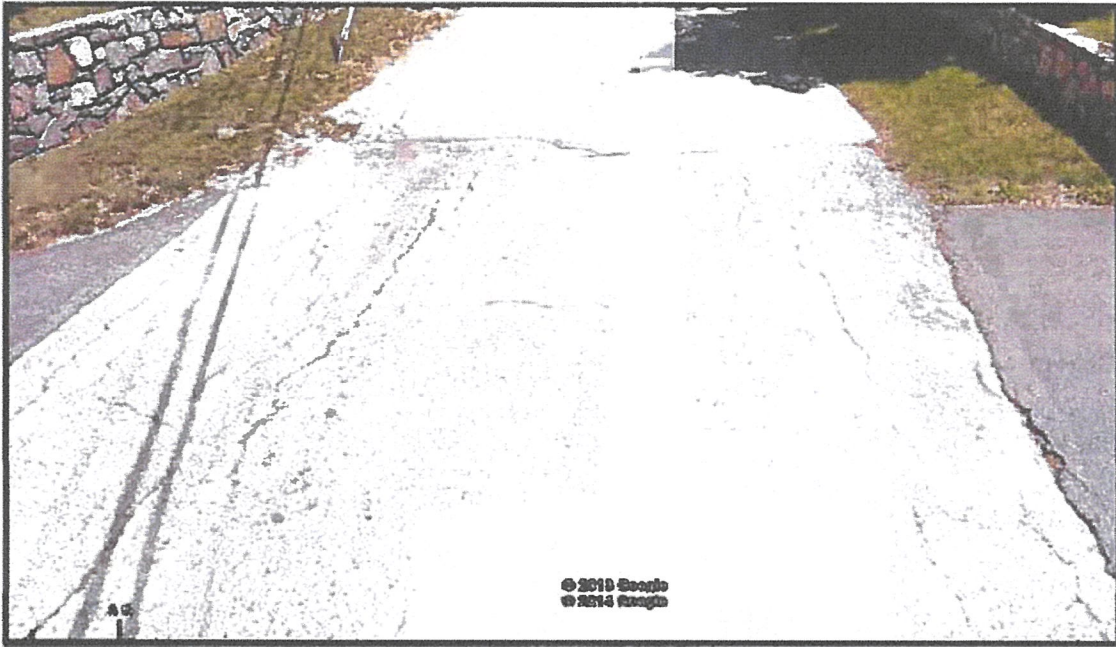
*Edge and Longitudinal cracking on Weeks Street, North Smithfield, RI.
