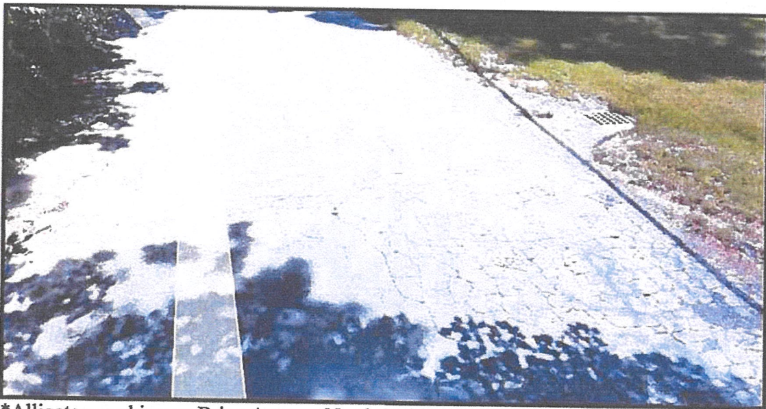
*Alligator cracking on Brian Avenue, North Smithfield, RI.
