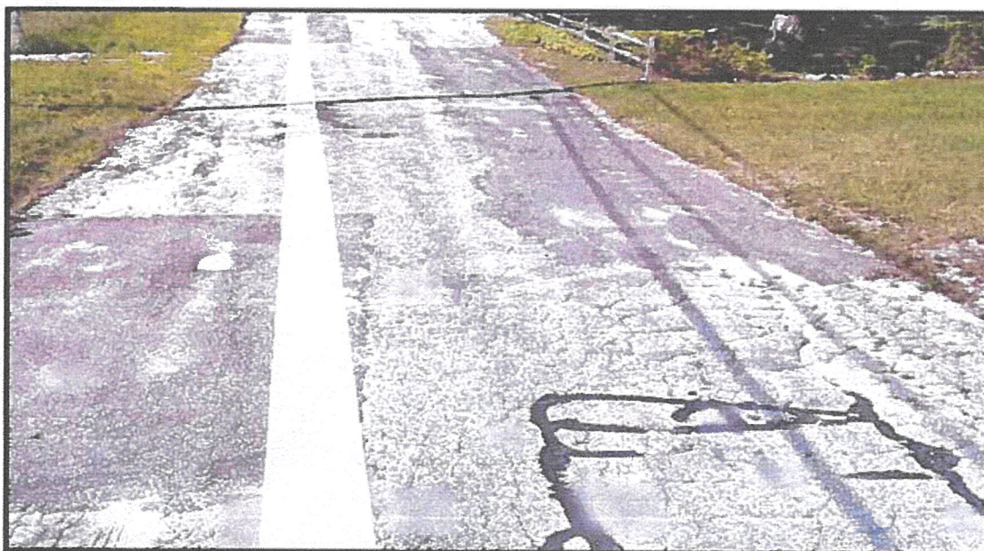
*Patching, Edge, Alligator cracking on Merrimac Road, North Smithfield, RI.
