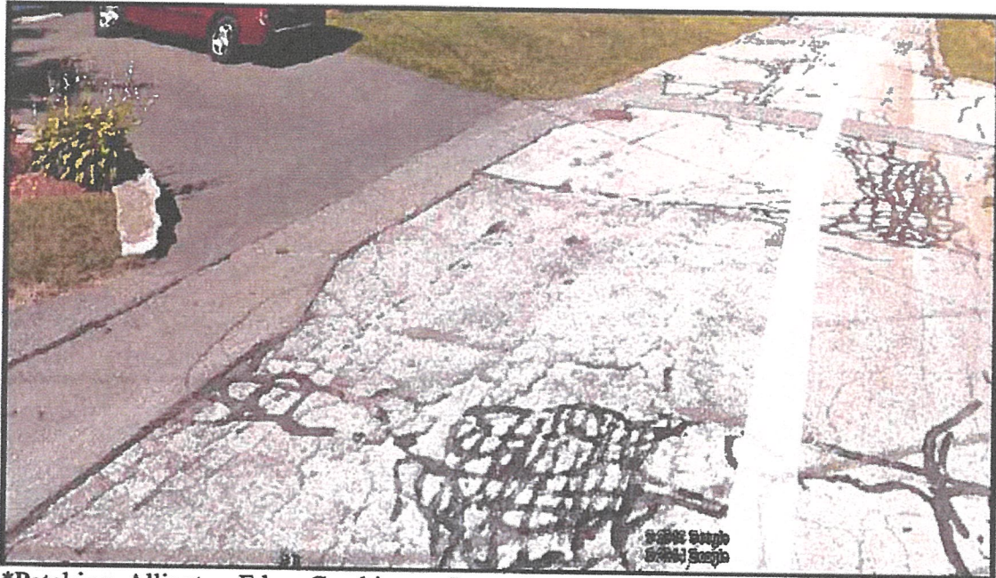
*Patching, Alligator, Edge, Cracking on Lapre Road, North Smithfield, RI.
