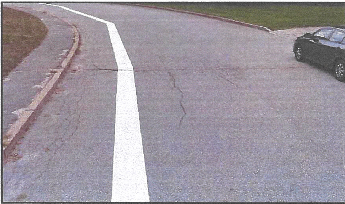
* Edge and Transverse cracking on Indigo Farm Road
