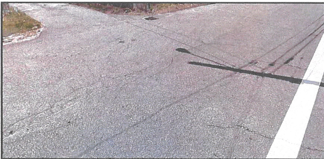
*Minor Alligator and Longitudinal cracking on Julie Avenue, North Smithfield, RI.
