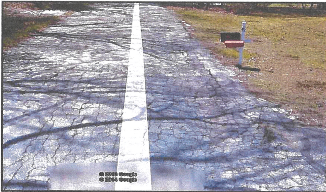
*Rutting and Alligator cracking on Carlton Avenue, North Smithfield, RI.
