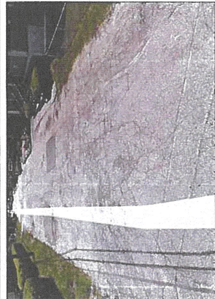
*SEVERE PAVEMENT DISTRESS ON MOWRY ROAD
