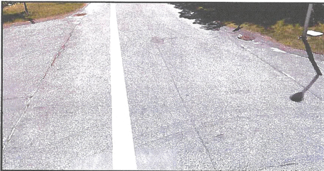
*Very minor Longitudinal Cracking on Bourget Court, North Smithfield, RI.
